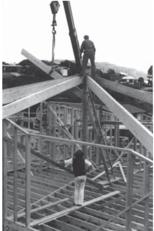
Paul Denford watching the central beam being lowered into place
