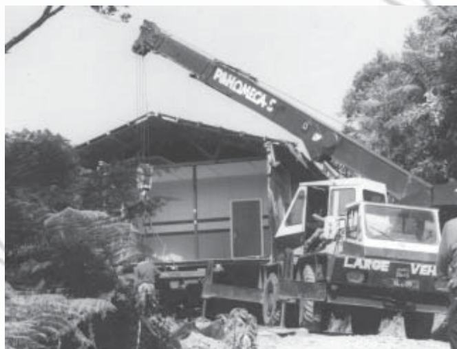
The buildings had to be craned around the corners
