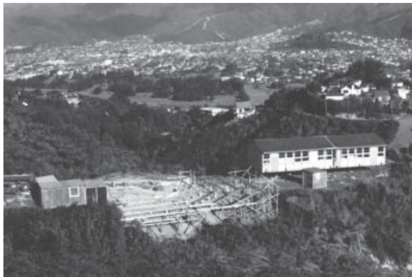
Moving the Class 1 and 2 prefab on site
